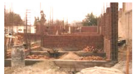
The walls go up
