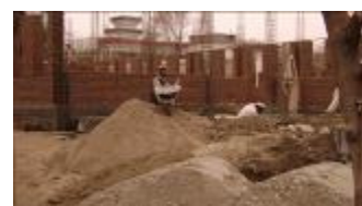
As more of the walls appear
